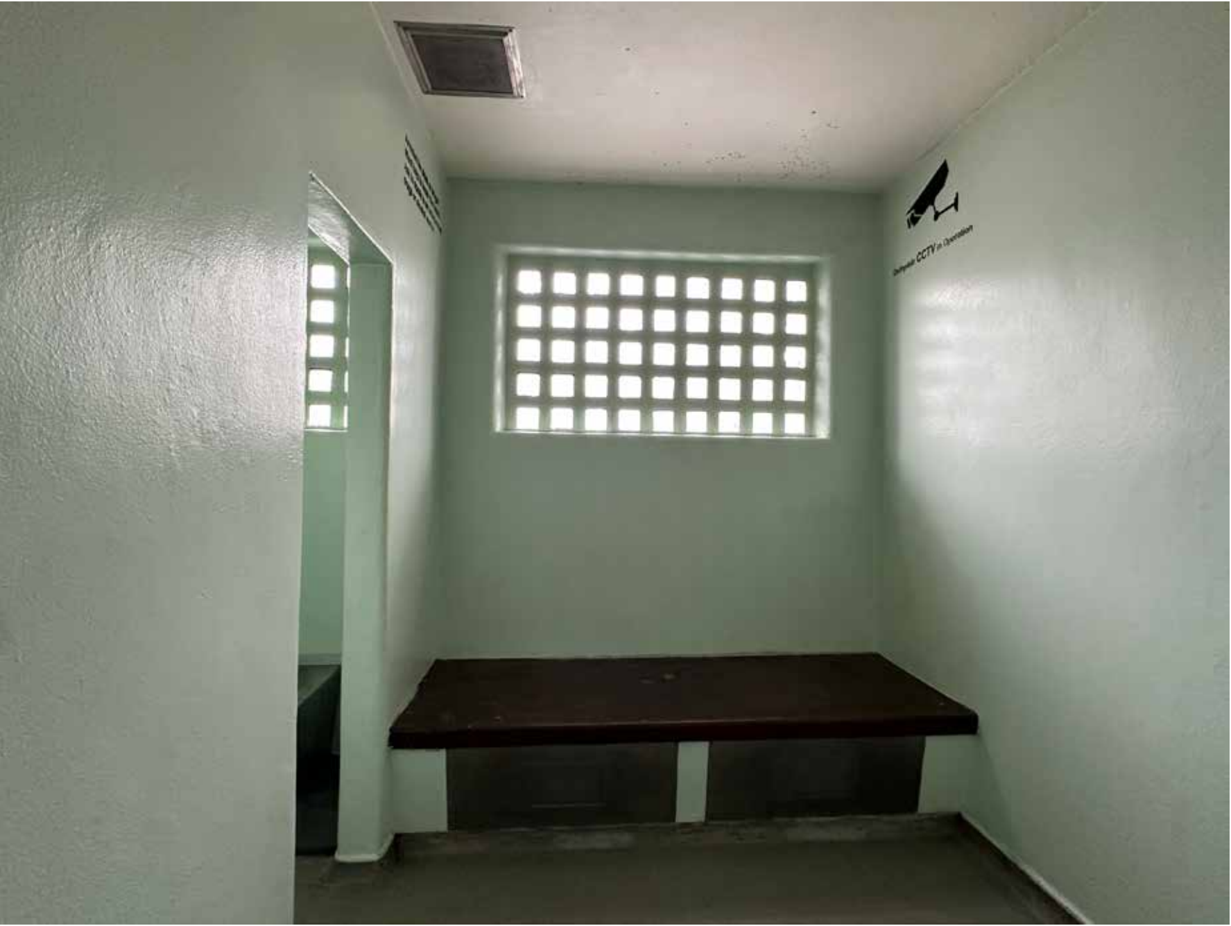
Existing prison cells - to be removed as part of the proposals - setting the 'community free'. A cell now replaced with a space for conversation and faith
